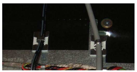
FIGURE 25 CABLE CLIPS HOLDING CABLES IN PLACE
